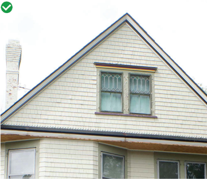
Original lead came windows intact and maintained
