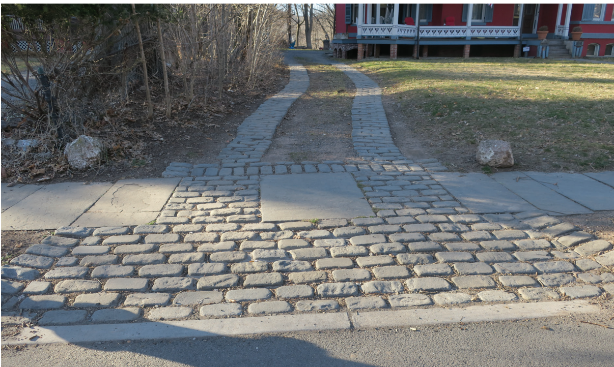
Historically appropriate driveway on Rockview Avenue residence property
