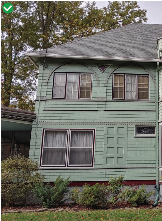
Concealed wire mast blending with house
