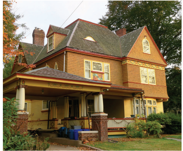
Asphalt shingle hipped roof with dormers
