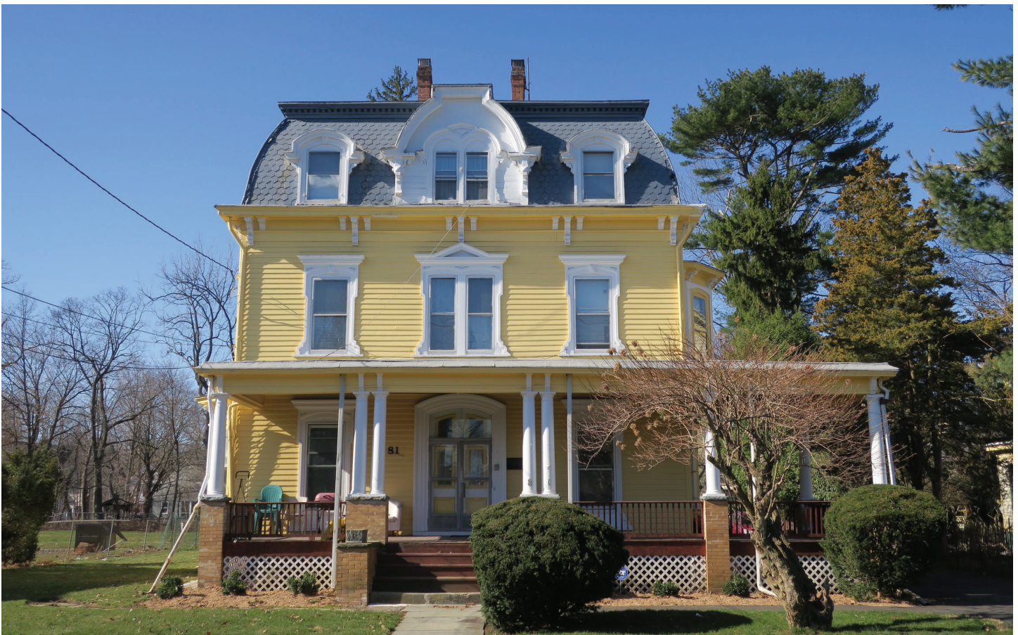
Grove Street residence
