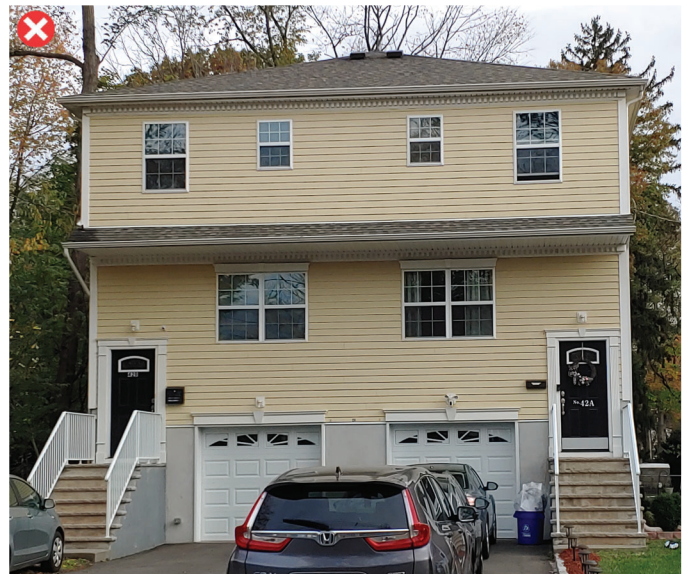
New construction with historically incompatible attached garages
