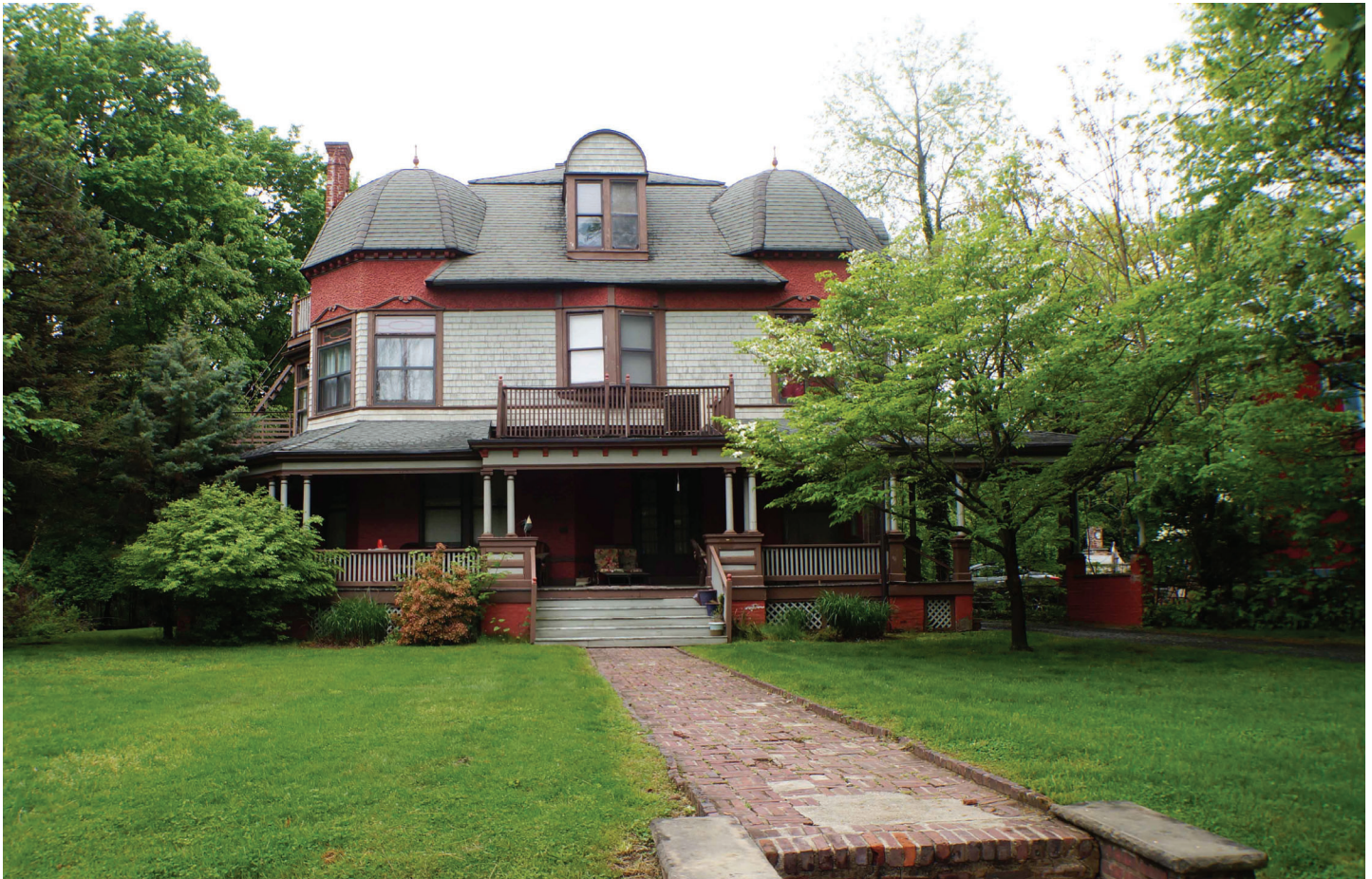
Rockview Avenue residence with historic brick walkway. Repairs to damaged areas should be made with in kind material
