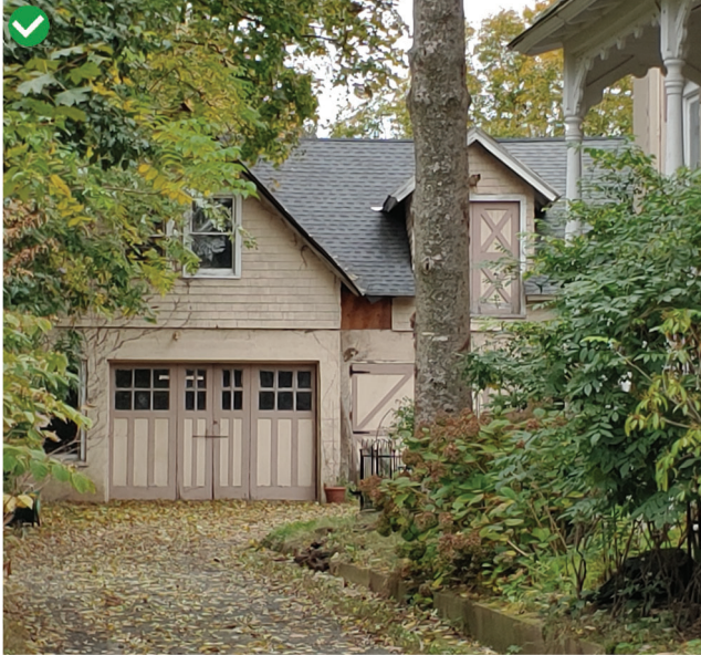
Well-maintained original carriage house
