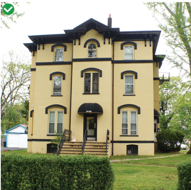
This textured stucco siding is in good repair with details appropriately highlighted
