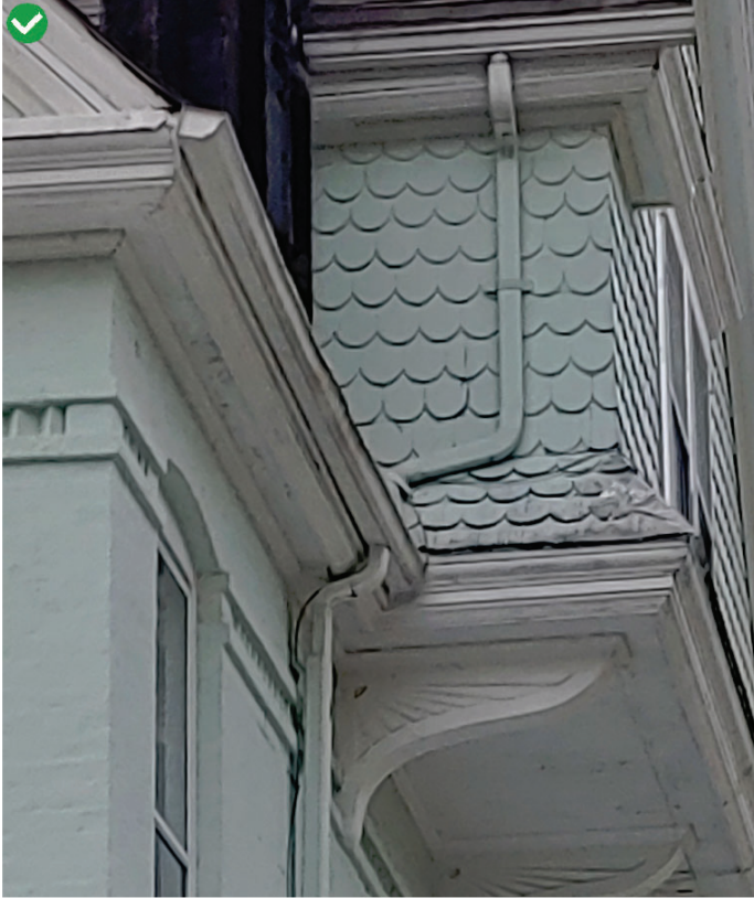
Downspout is concealed and matches shingle paint.
