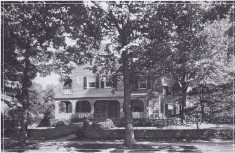
RESIDENCE OF WALTER M. MCGEE, 101 ROCKVIEW AVENUE
