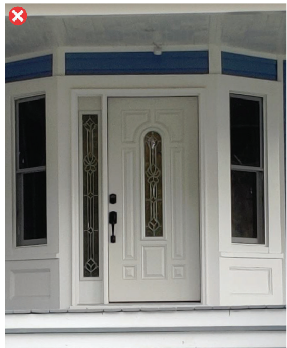
Modern fiberglass with sidelight
