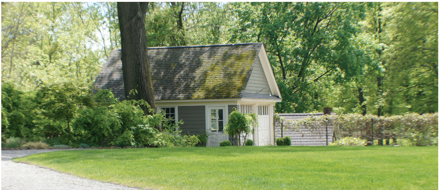
Garage on Rockview Terrace property
