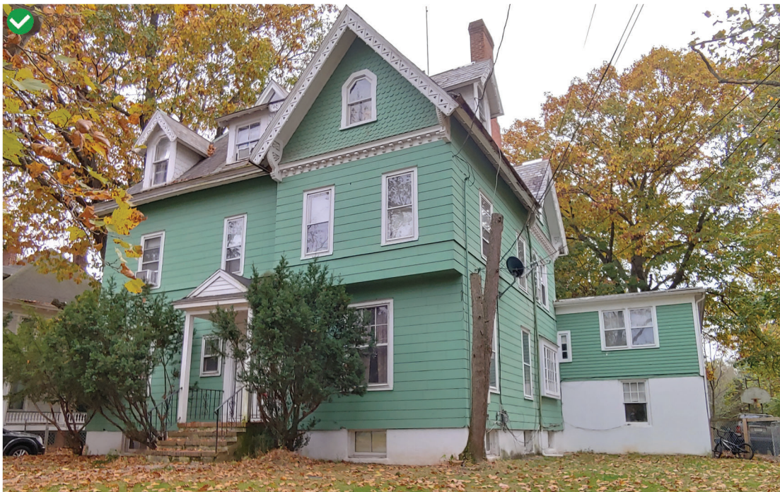
Rear yard garage addition matches paint color with differentiated clapboard
