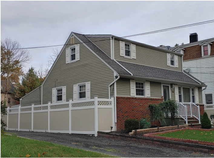
Asphalt shingle side-gable with dormer
