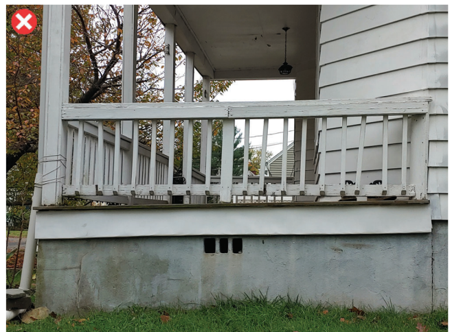
Foundation infilled with concrete block
