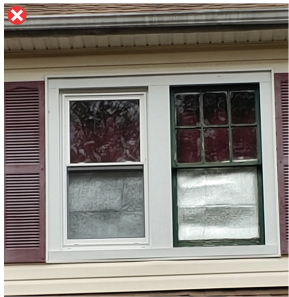
Replacement aluminum window (left) and original wood window (right)
