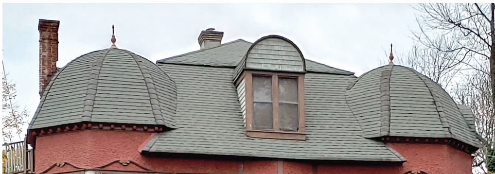
Asphalt shingle roof with towers and dormers
