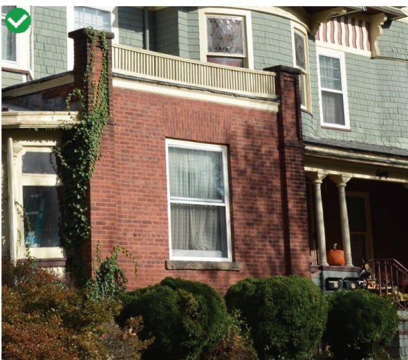
Brickwork maintains its original intent and appearance
