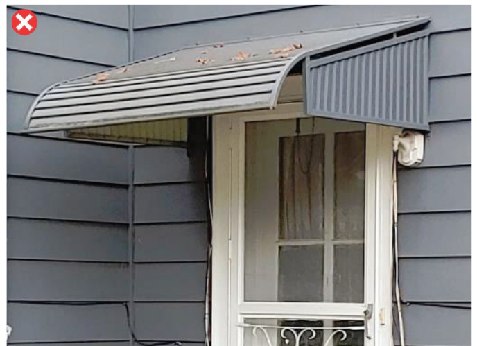
Sheet metal awning
