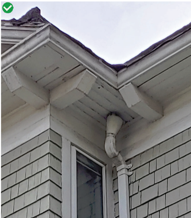
Downspout placement underneath roof fascia
