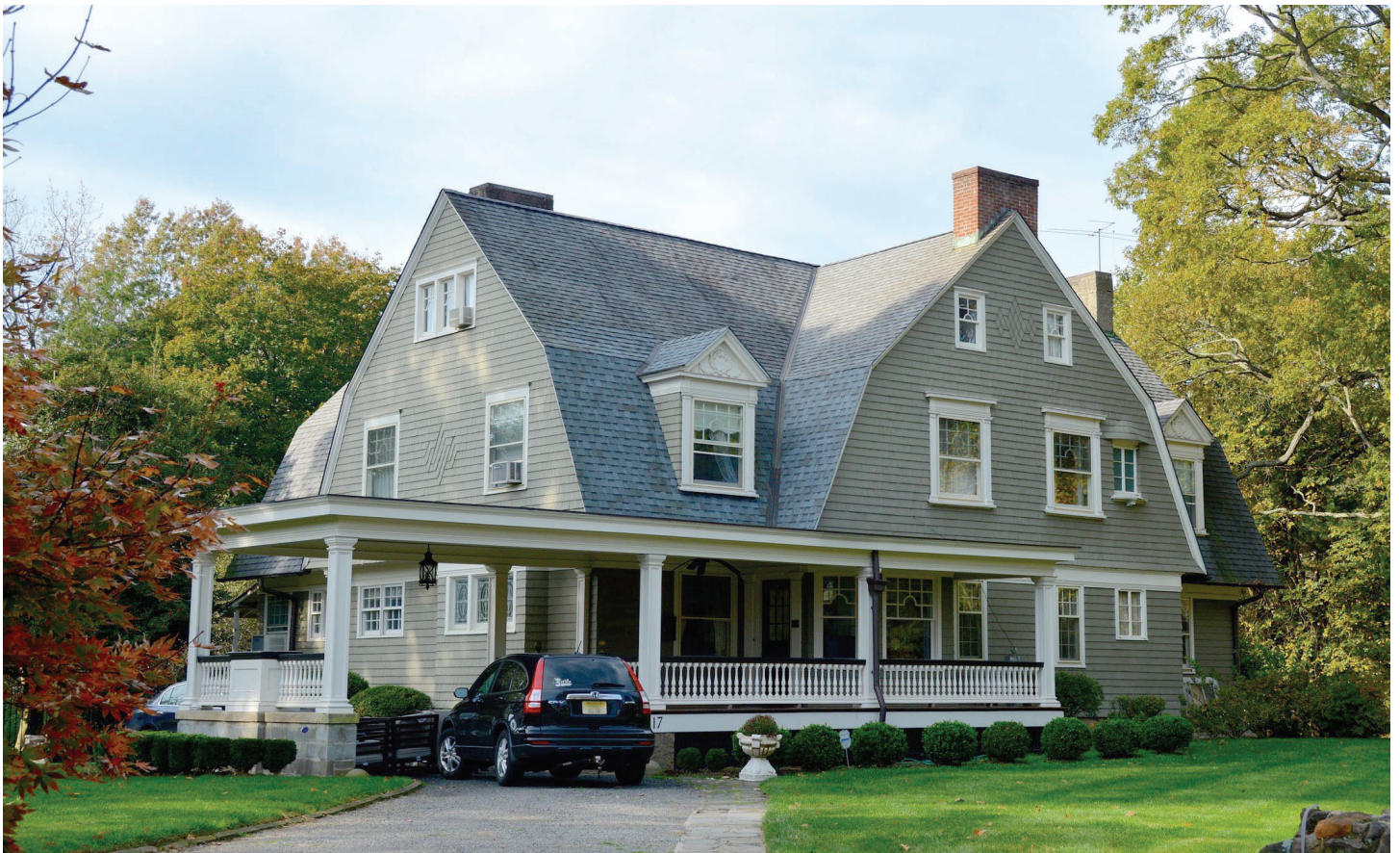
Shingle Style residence, Rockview Terrace
