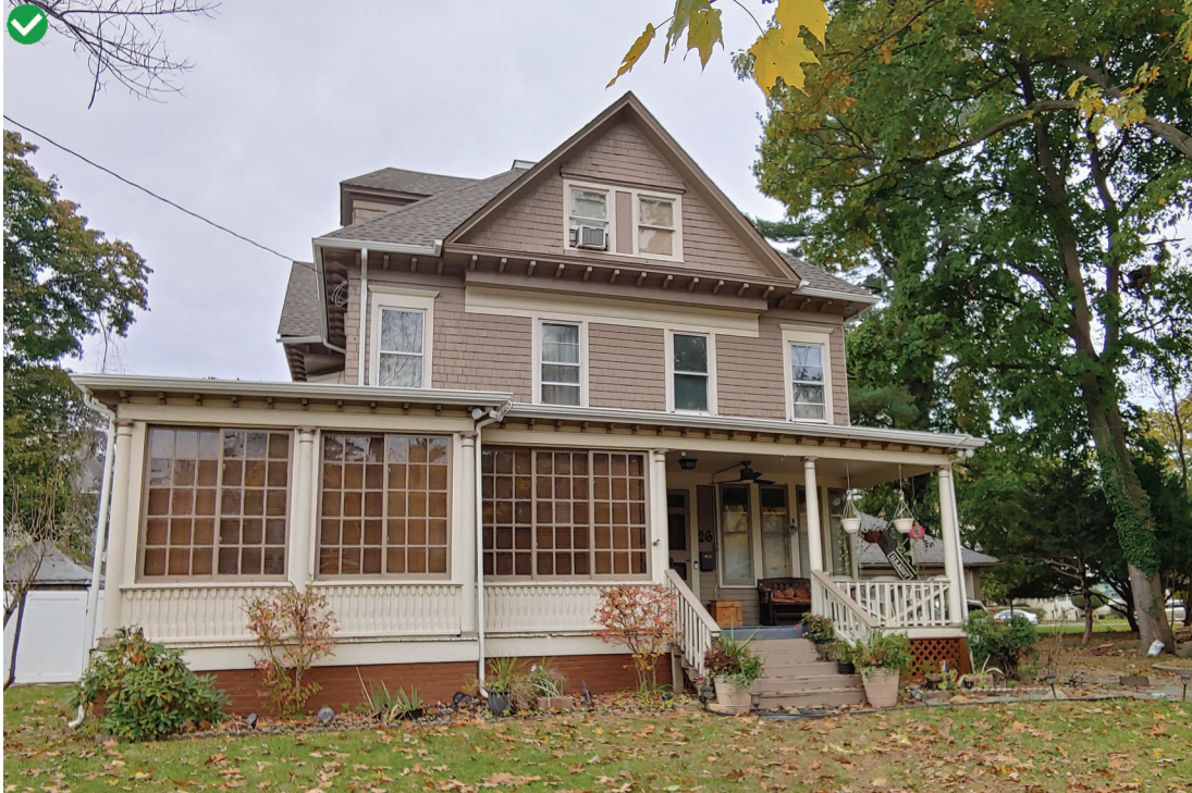
Partial front porch enclosure compatible with original building
