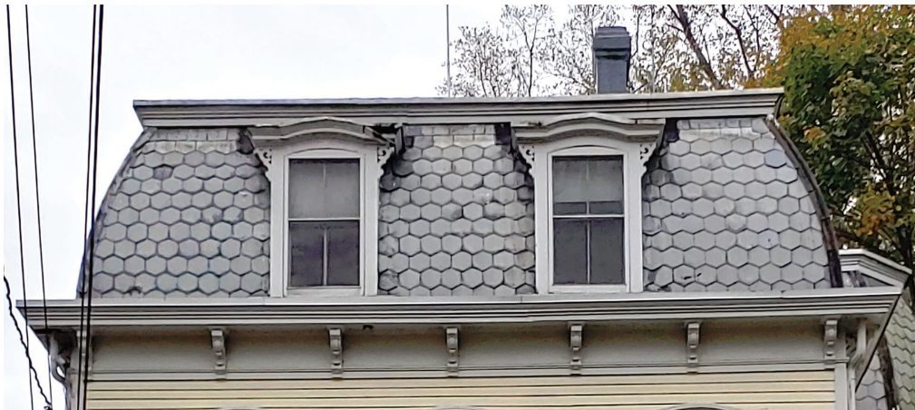
Convex mansard with slate shingles
