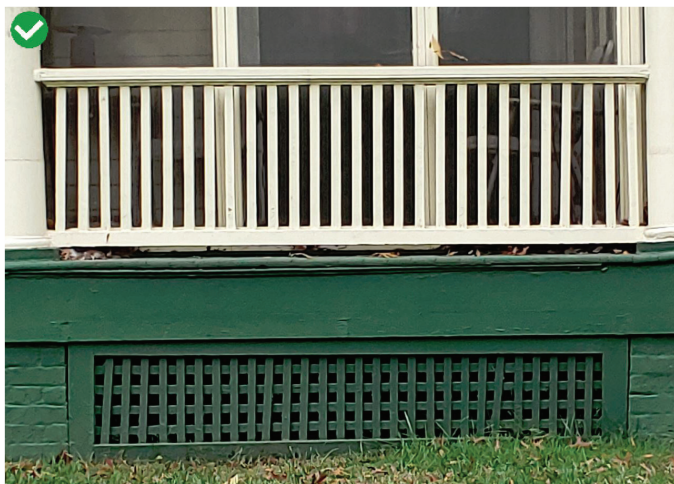
Wood lattice panel infill
