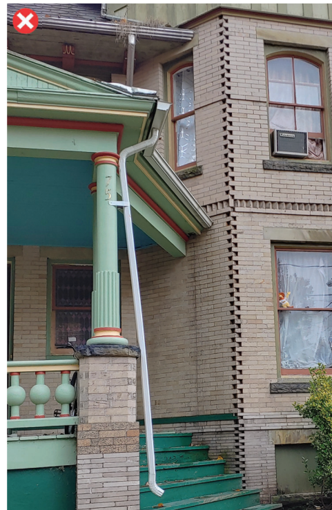
Downspout placement outside of cornice
