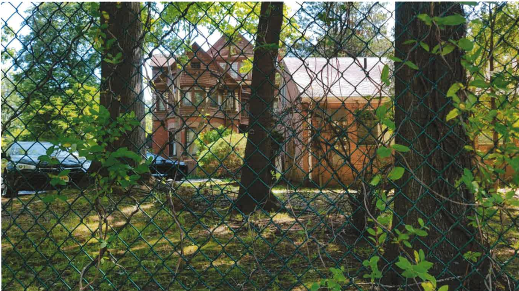
GROUND VIEW OF EXISTING PERIMETER FENCE TO BE REPLACED WITH DECORATIVE FENCE (TAKEN BY JOHN MCDONOUGH ASSOCIATES ON MAY 31, 2023)
