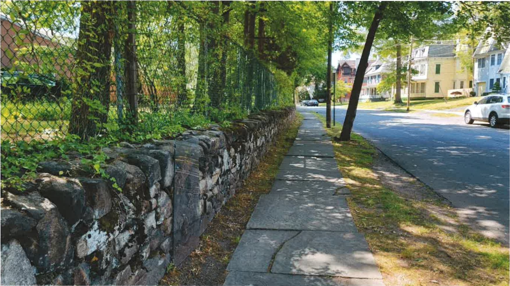
GROUND VIEW OF EXISTING PERIMTER FENCE TO BE REPLACED WITH DECORATIVE FENCE (TAKEN BY JOHN MCDONOUGH ASSOCIATES ON MAY 31, 2023)
