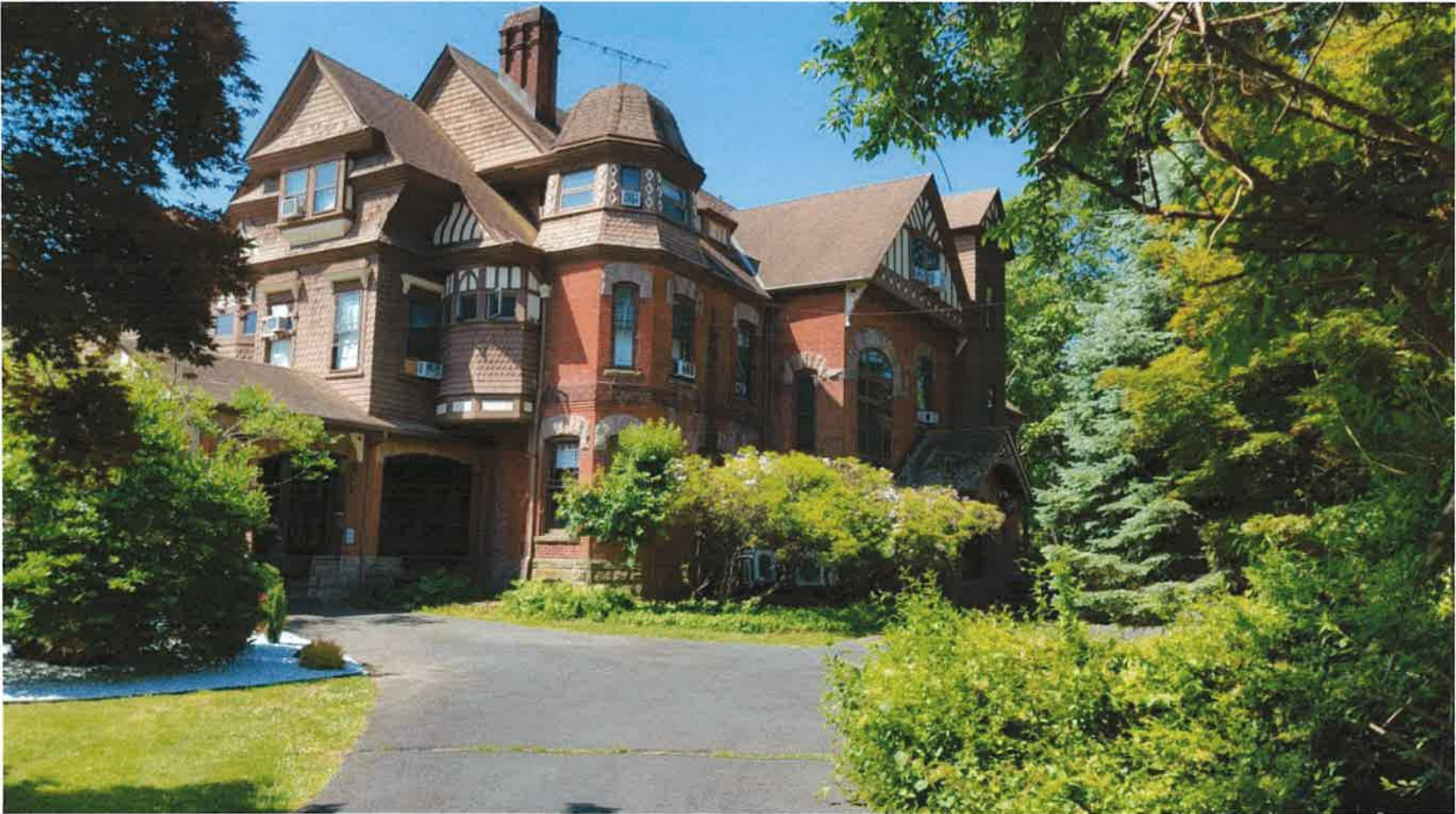
GROUND VIEW OF CENTERPIECE HISTORIC MANSION PRESERVED AND ADAPTIVELY RE-USED (TAKEN BY JOHN MCDONOUGH ASSOCIATES ON MAY 31, 2023)
